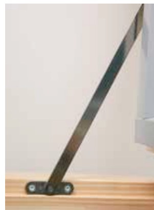
Handle operated hold open friction stay for SHI.
